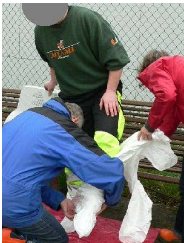
Fig. 3.22 Putting on the coverall. The worker is wearing Tyvek™ shoe covers over his work shoes to avoid contamination.
