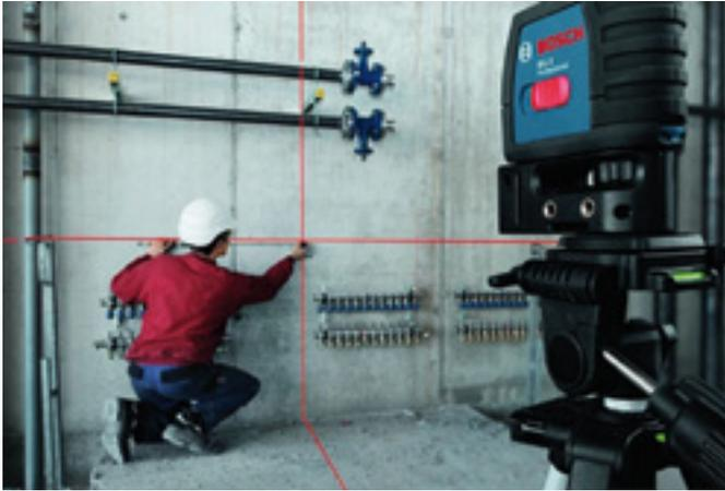
**Figure 6** An alignment laser
